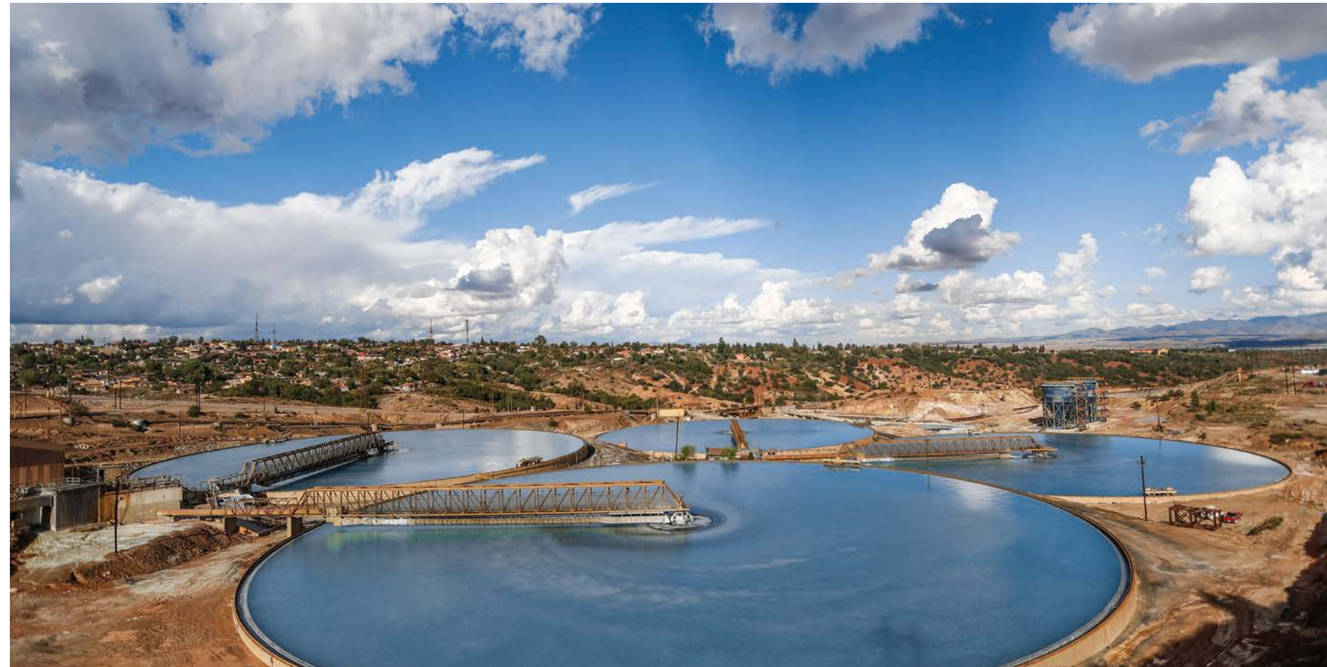
The different mineral processing processes produce tailings, containing water and solids that are passed through thickeners where most of the water is recovered.
