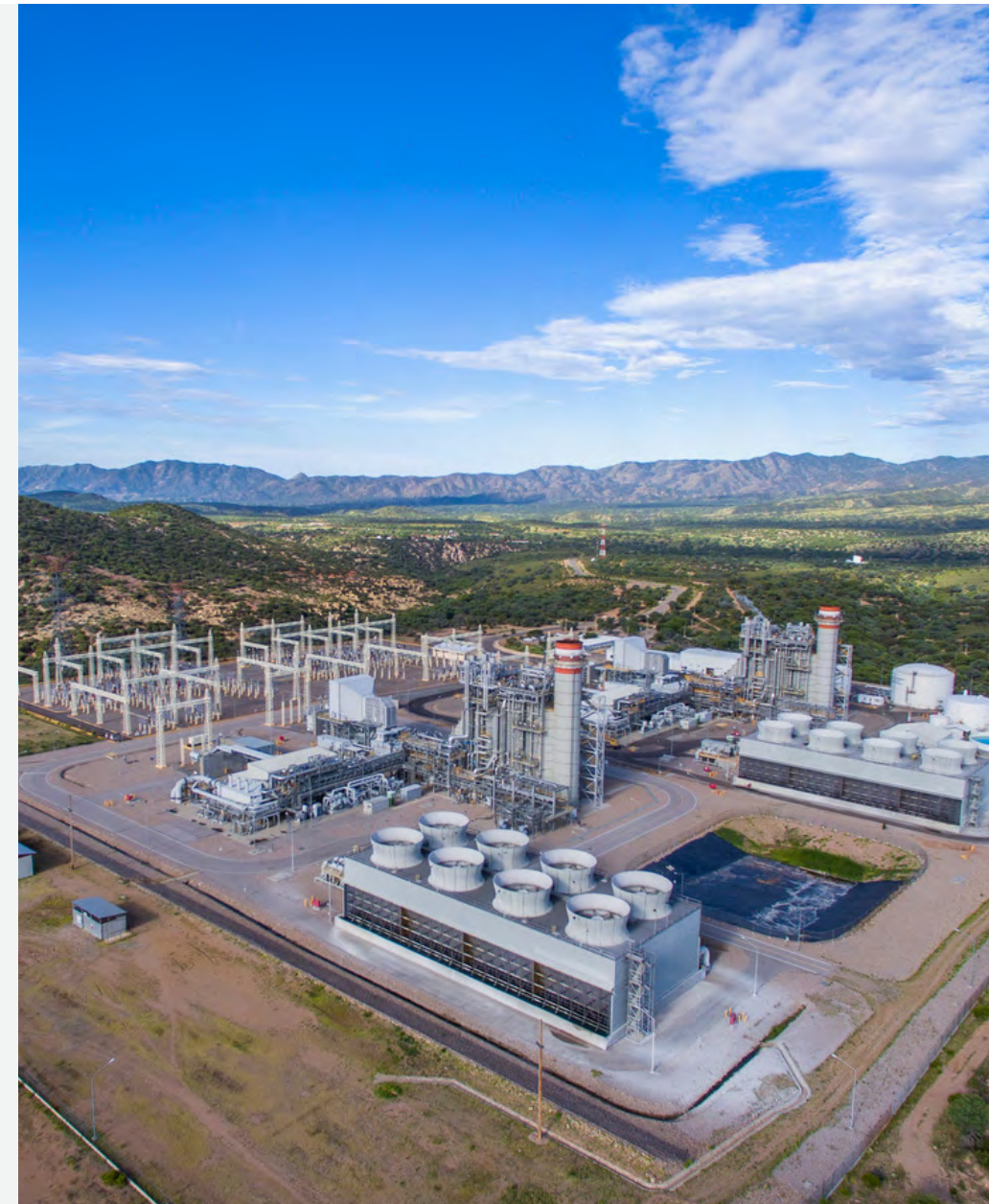
📷 Combined Cycle Plant in Nacoziari de García, Sonora, Mexico.
