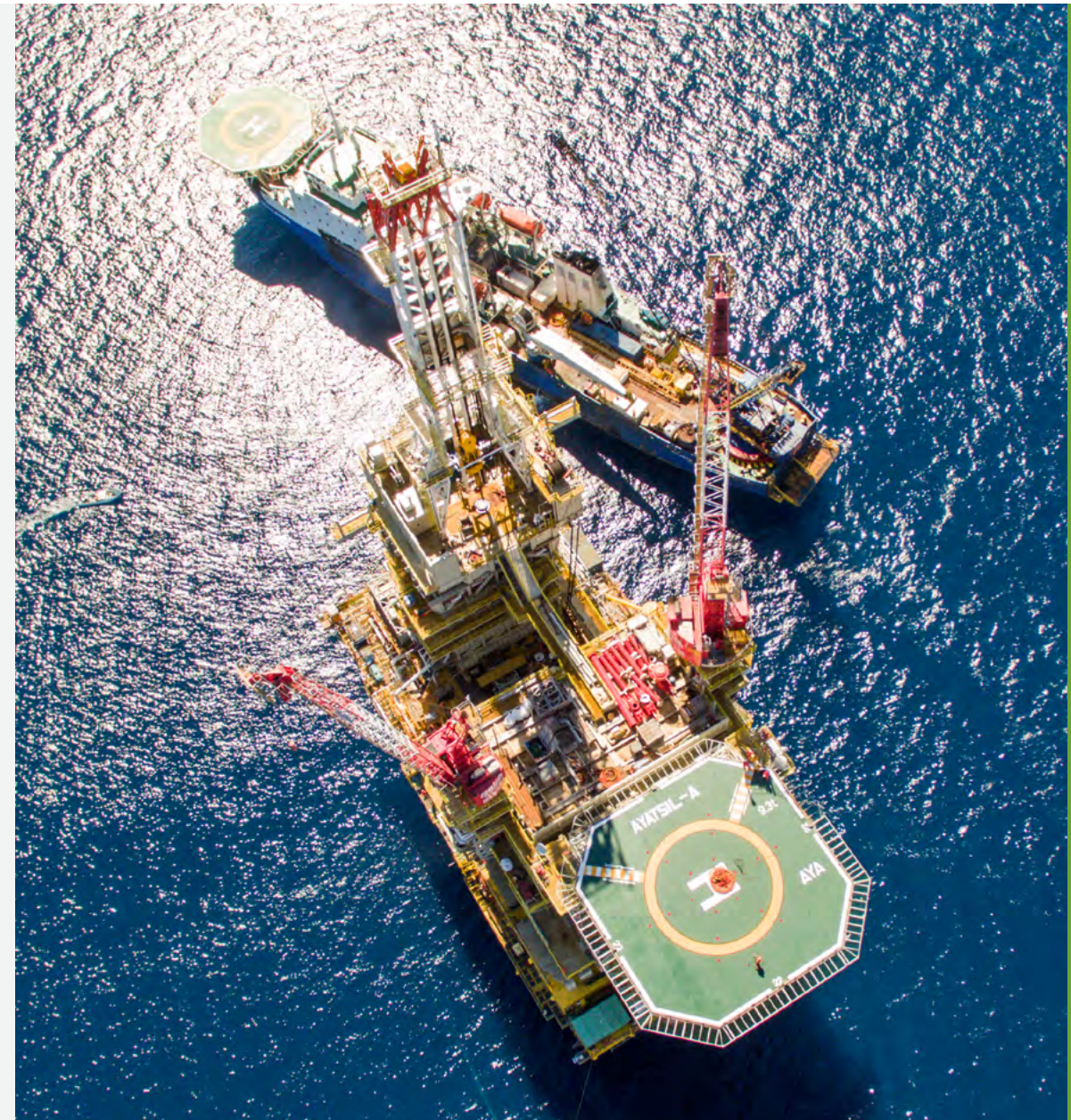
Perforadora México's Veracruz Lifting Platform in the Pacific Ocean, Mexico.
