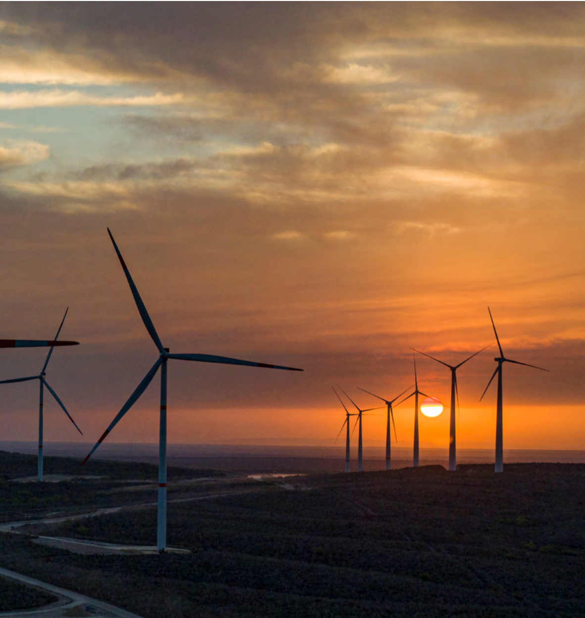
📷 New 168 MW Fenicias wind farm in northern Mexico.
